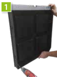
▪ Attach back frame to wall
